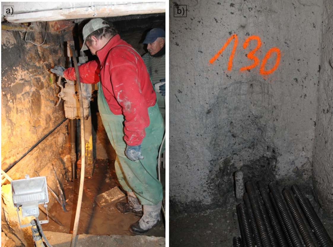
Fig. 8. Drilling of micropiles in the basement
